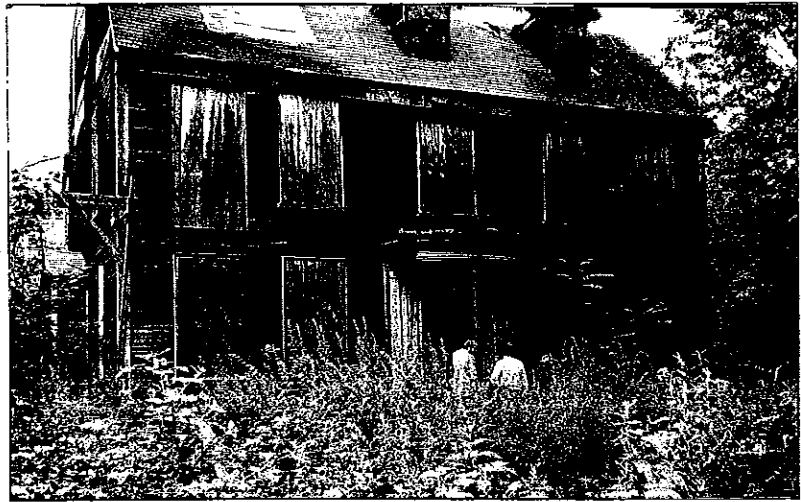
Before its recent restoration, the Dillaway-Thomas House in Roxbury was a burned-out hulk.
